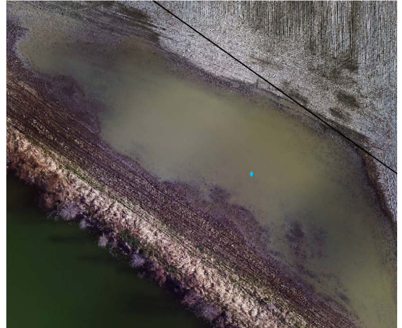
Seepage behind dike
